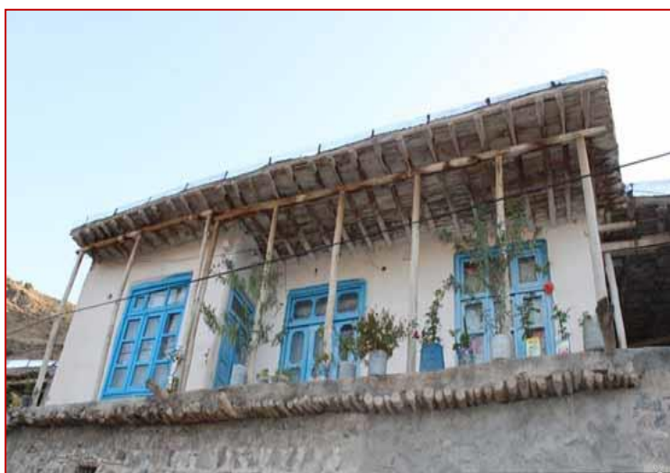
Main façade a house in Kazaj village plastered with Alava material.
